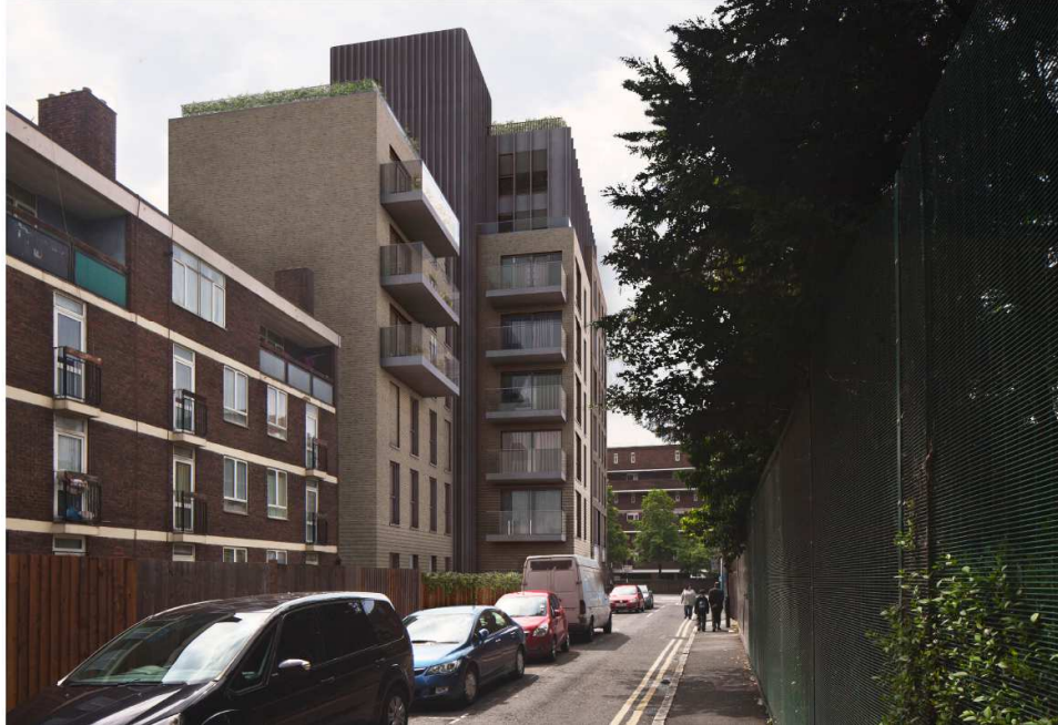
Figure 5 - View south towards Commercial Road
