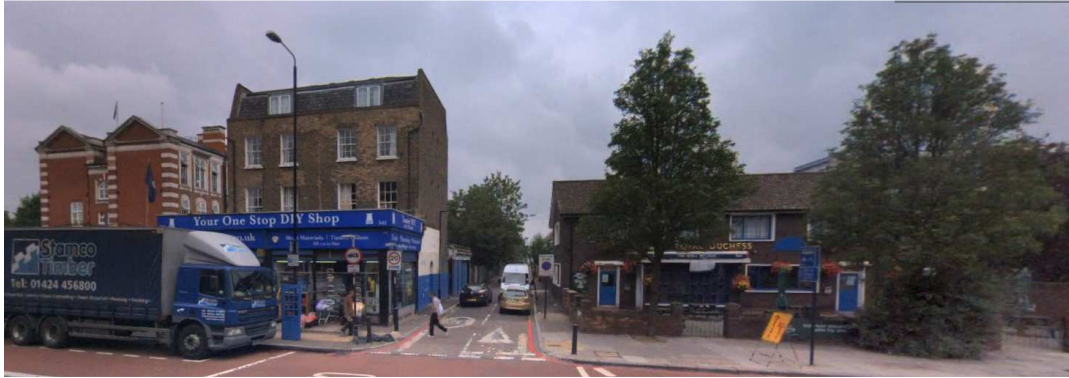
Figure 2 - The application site (Public House now demolished), narrow Head Street and corner building
